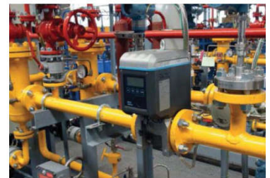
Gas flow measurement in municipal utilities: FLOWSIC500 with integrated flow conversion
